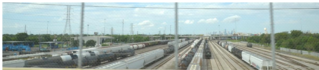
Union Pacific rail tracks, Houston. (OIG photo)
