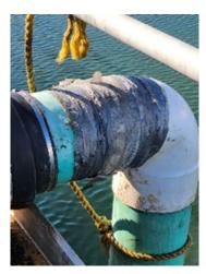
Example of poor maintenance of pipes using duct tape at the traditional side of the OB Curtis plant. (EPA OIG photo)
