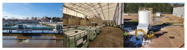
Left to right: O.B. Curtis conventional water treatment, liquid soda ash storage and membrane treatment, and external liquid lime treatment tank. (EPA OIG images)
