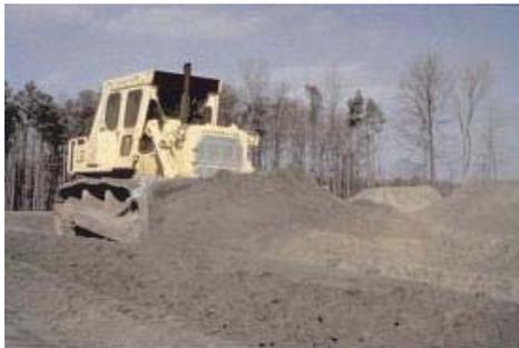
Spreading and compacting fly ash structural fill. (EPA photo)
