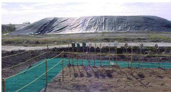
The contaminated soil mound contained within a high density polyethylene cap at the Escambia Treating Company Superfund site (EPA OIG photo).
